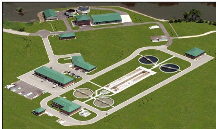
Aerial view of the Watertown WWTP
