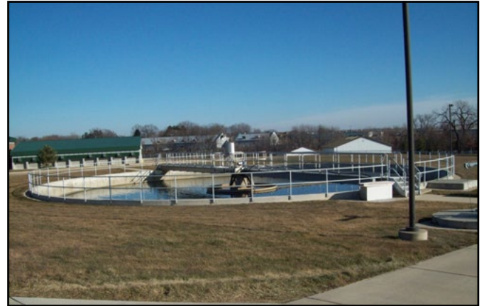
The City of Watertown Wastewater Treatment Plant
